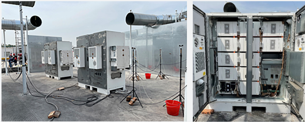
Figure 17. Multiple observation devices used to accurately capture test results Left: test site layout; Right: tested cabinet
